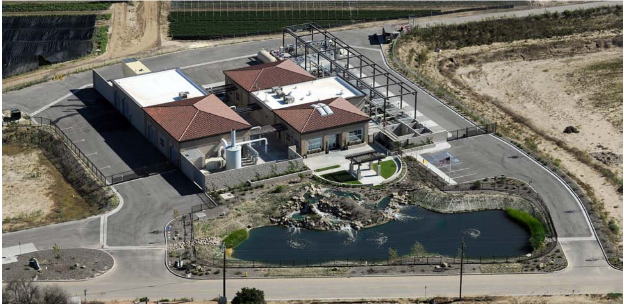
The Santa Paula (Calif.) Water Recycling Facility, originally anticipated to reduce energy consumption by 15%, now is more than 35% energy-efficient than the city's original wastewater treatment plant. Craig Mailloux
