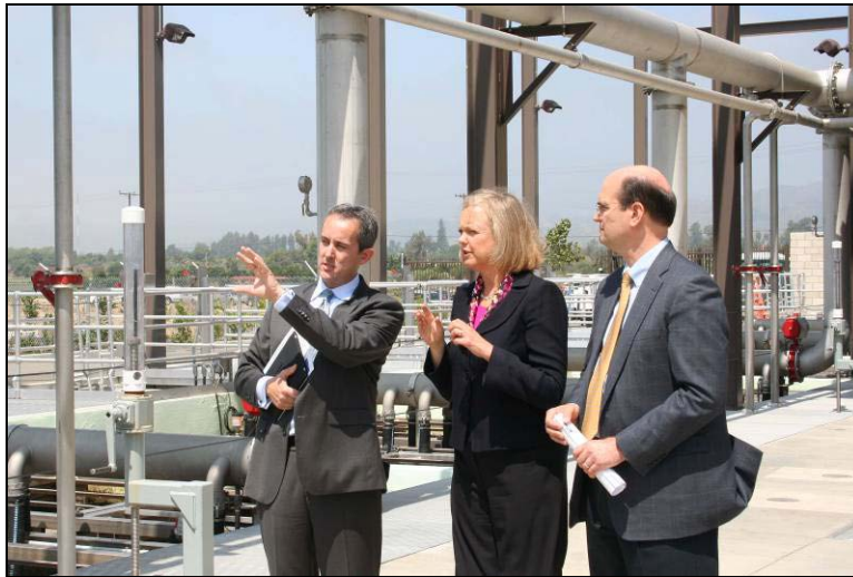
Brian Cullen (PERC Water), Meg Whitman (CA Gubernatorial Candidate) and Phil Dyk (Alinda Capital) tour Santa Paula Water Recycling Facility.
