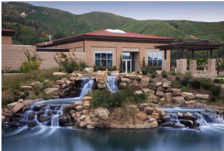
The Santa Paula Water Recycling Facility
