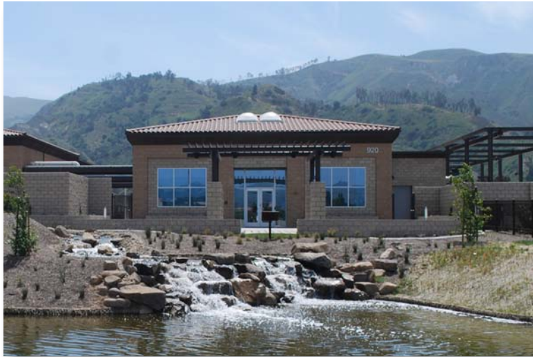
Santa Paula Water Recycling Facility
