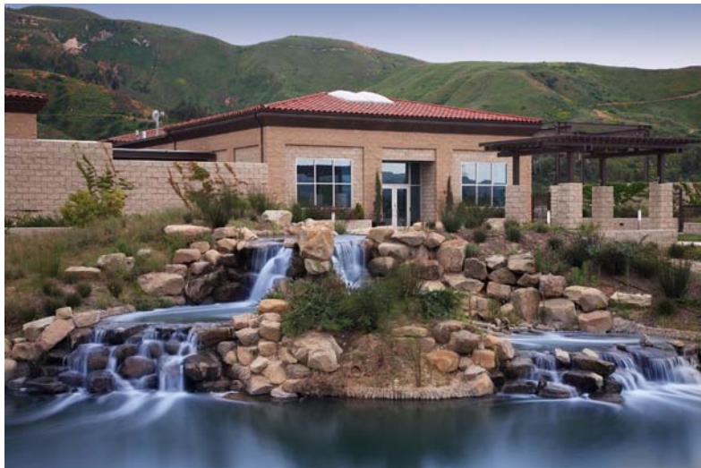
Santa Paula Water Recycling Facility, Ventura County, California
