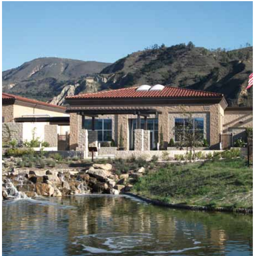
The Santa Paula Water Recycling Facility in California
